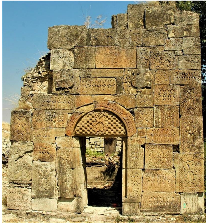
Figure 6 The facade of the small church of Bri Eghts Monastery. Photo: H. Petrosyan.
